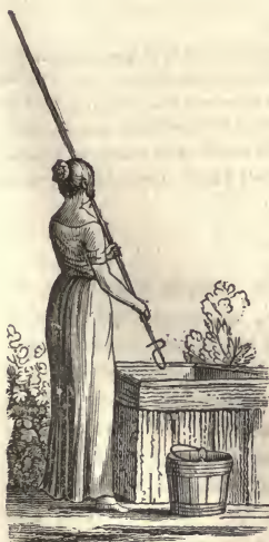
No. 10. Cistern Pole.
